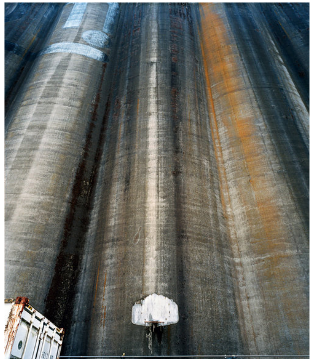
Grain silo, Portland, Oregon; 2007.
